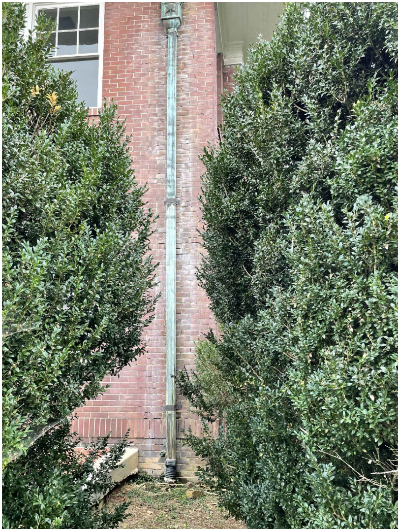
Repoint brick in the area damaged by water at downspout.
