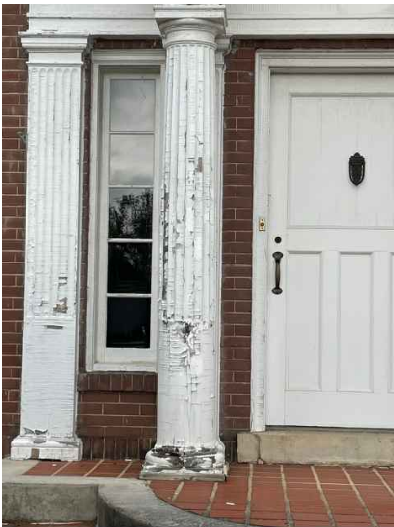
Repair, reglaze, and paint sidelights. Repair existing columns as noted on sheet A1.2.
