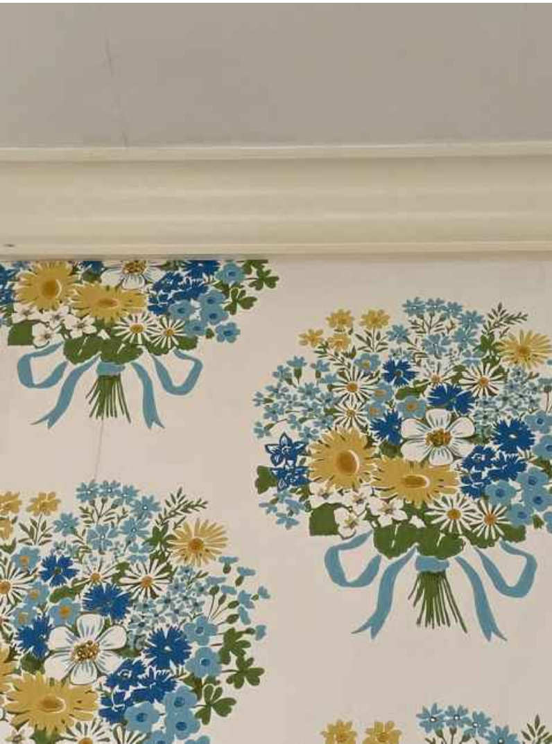
All walls with existing wall covering shall be cleaned, primed, and painted (two coats, eggshell premium grade latex paint). Walls, ceiling, base board, and crown molding is to be painted.
