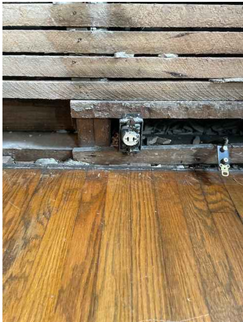
Plaster has been removed; therefore, contractors can see the existing wall framing.
