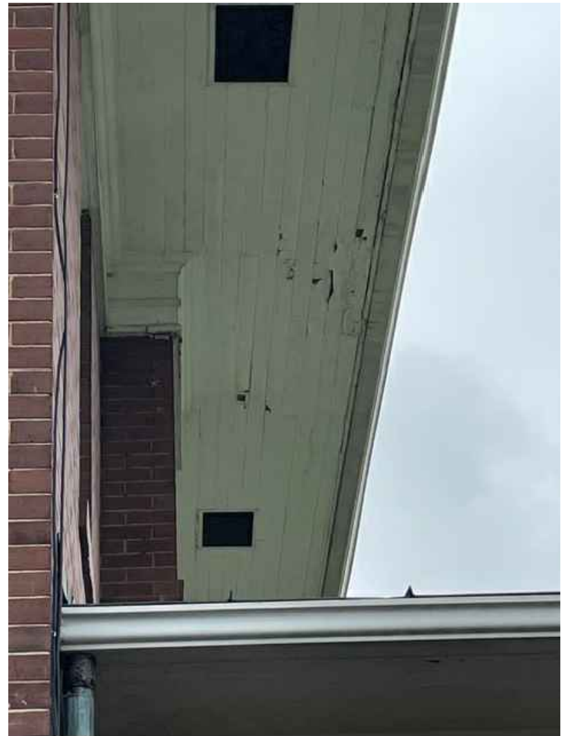
Remove and replace all damaged soffit and fascia. Paint soffit, fascia, and trim.
