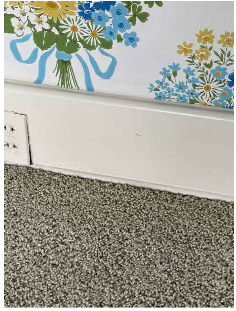
All walls with existing wall covering shall be cleaned, primed, and painted (two coats, eggshell premium grade latex paint). Walls, ceiling, base board, and crown molding is to be painted.
