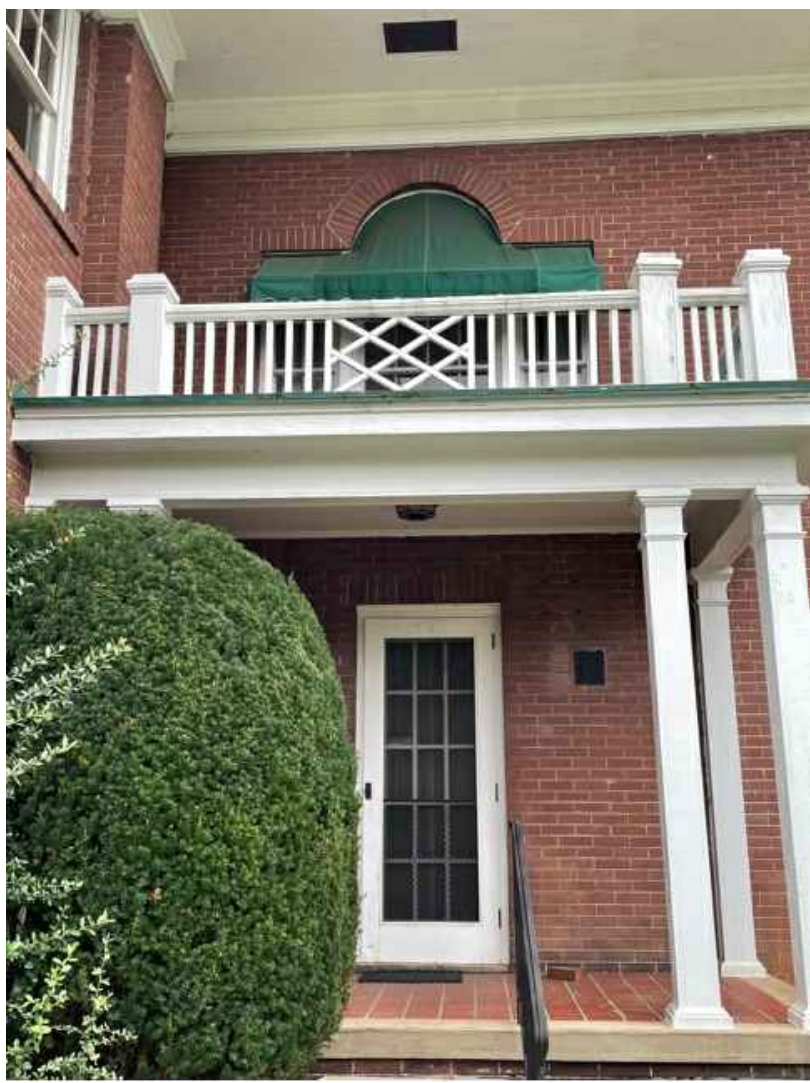
Remove existing railing on porch roof. Replace with composite materials of the same size (railings, post, post cap, post base, balusters, etc...) Upon removal, contractor shall verify dimensions, details, and attachment metal to roof structure below.
