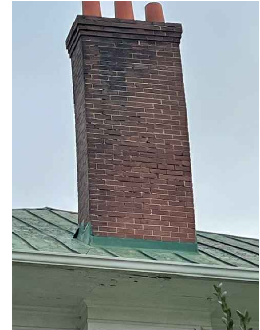
Remove and replace all damaged soffit and fascia. Paint soffit, fascia, and trim. Repoint chimney.
