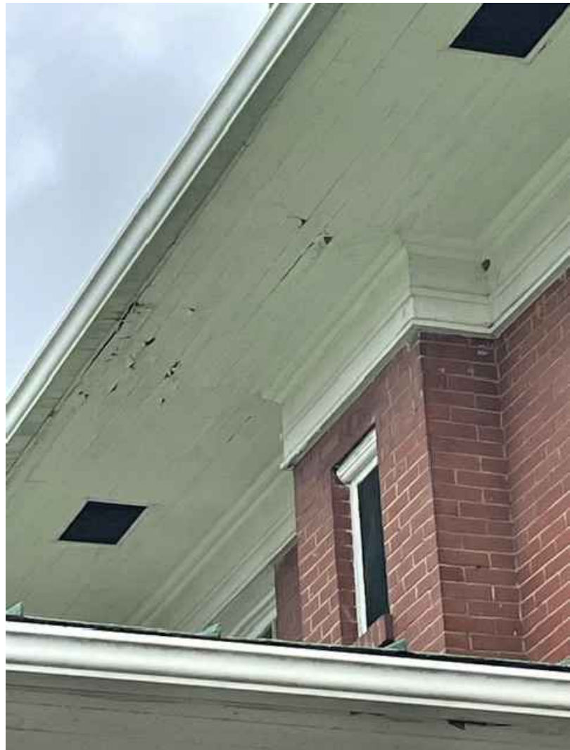
Remove and replace all damaged soffit and fascia. Paint soffit, fascia, and trim. Small window is to be repaired, reglazed, and painted.
