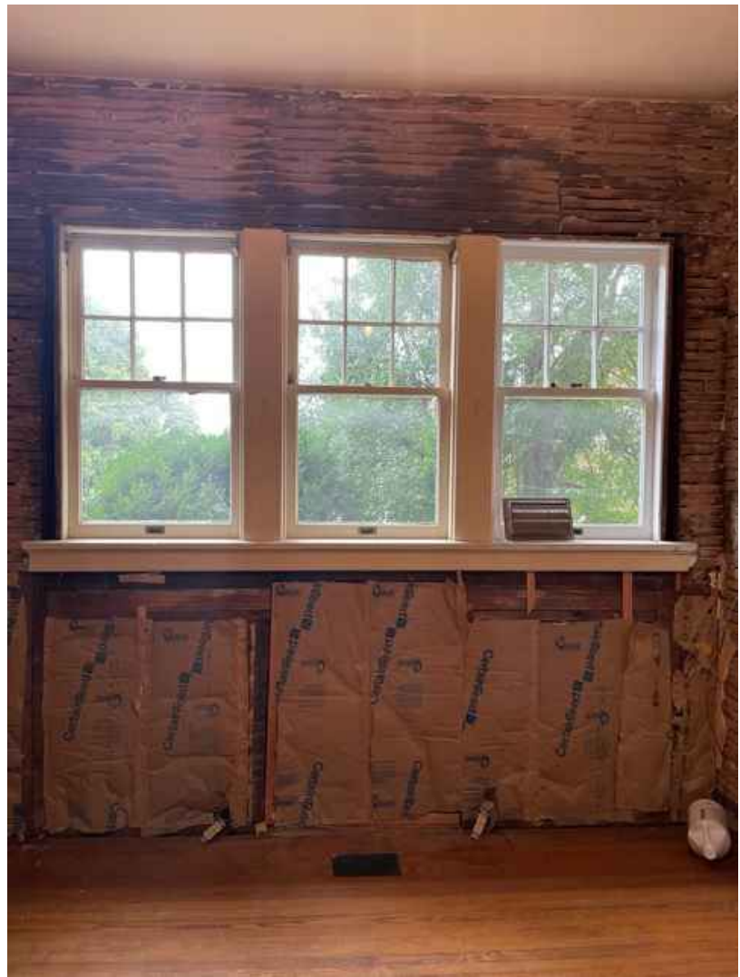
Windows to be replaced wood windows with matching size and style. Plaster has been removed; therefore, contractors can see the existing wall framing.
