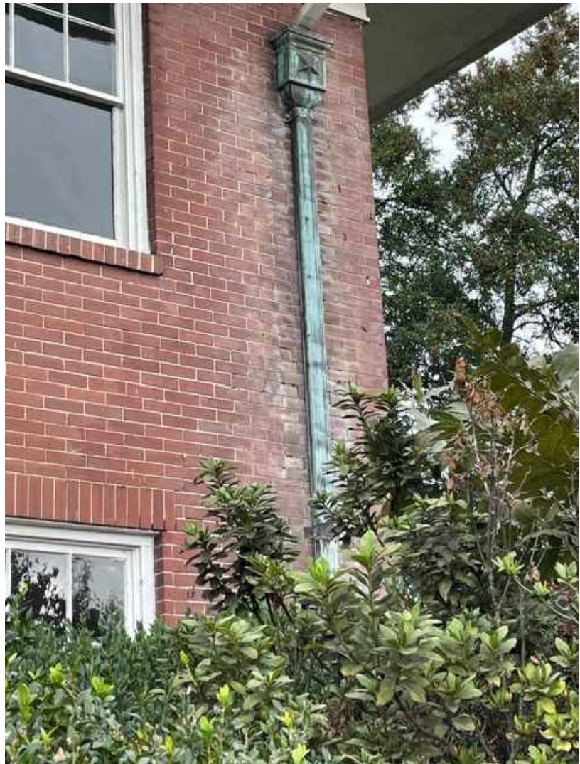
Repoint brick in the area damaged by water at downspout.
