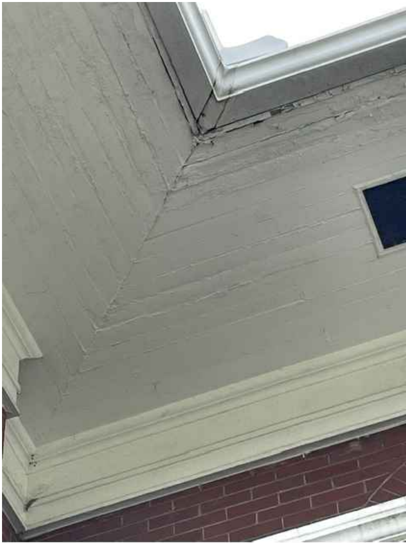
Remove and replace all damaged soffit and fascia. Paint soffit, fascia, and trim.
