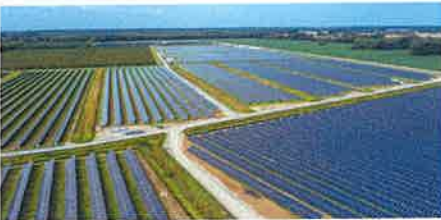
Altavista Solar (80 MW) Lynch Station, Virginia
