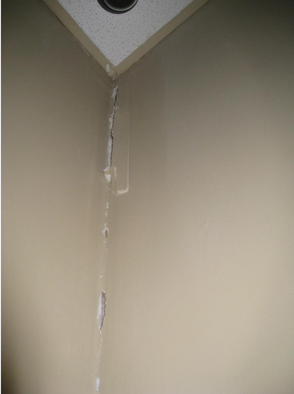
Picture 2: Crack in sheetrock at intersection of interior and exterior walls.
