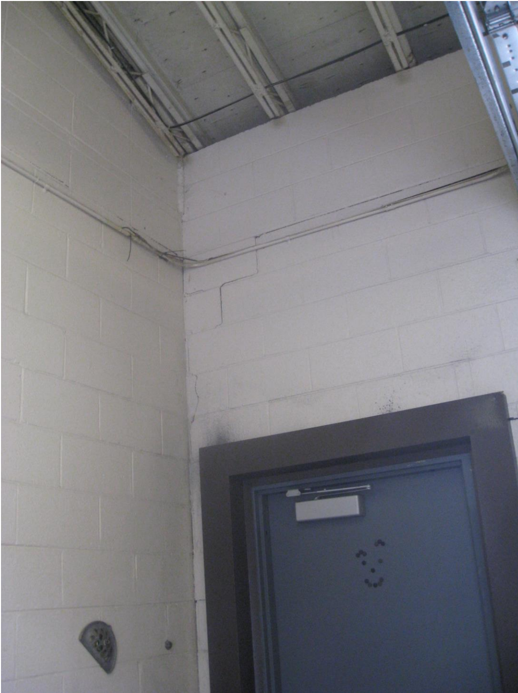
Picture 12: Settlement crack in the masonry of the Sally Port.
