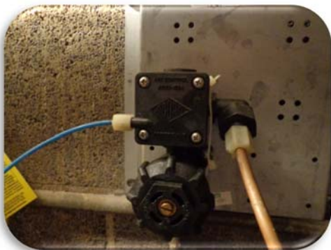
Acorn pneumatic actuated water valve for inmate sink
