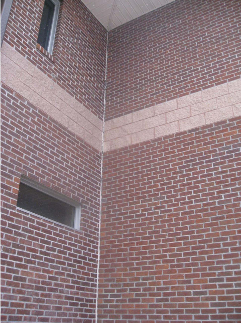
Picture 13: Exterior view of the separation of the newest stair tower from the building addition.
