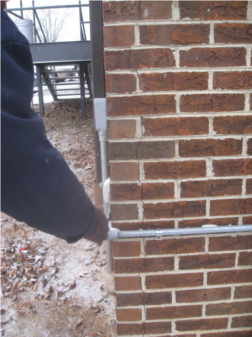
Picture 11: Corner cracks in brick due to lack of expansion joints in the veneer.
