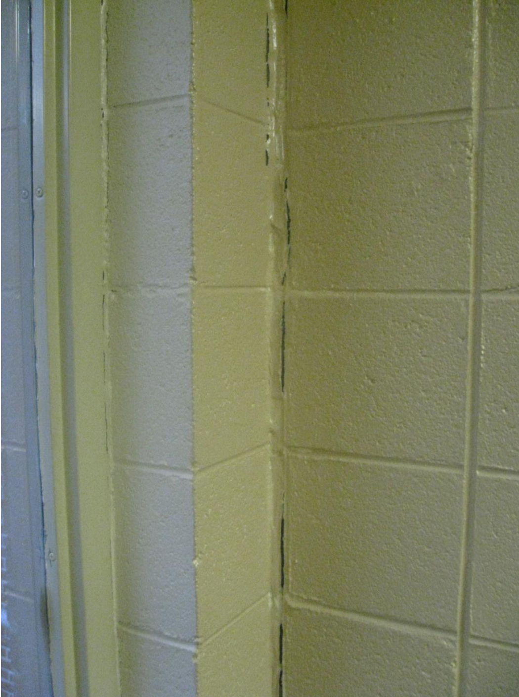
Picture 3: Separation of stack-bond masonry at intersection of interior and exterior walls.
