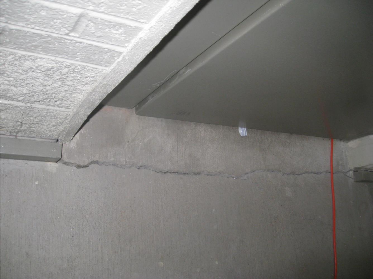
Picture 9: Crack in the second floor landing slab at the north stair tower of the addition..
