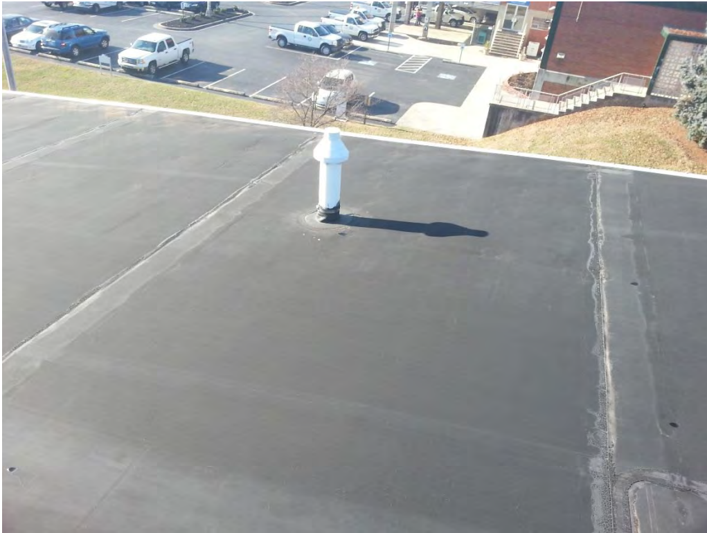
Vent above furnace. Maintenance on flashing needed.
