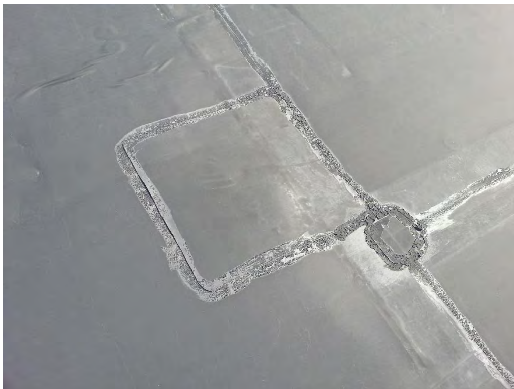
Seams beginning to curl and adhesive deteriorating.
