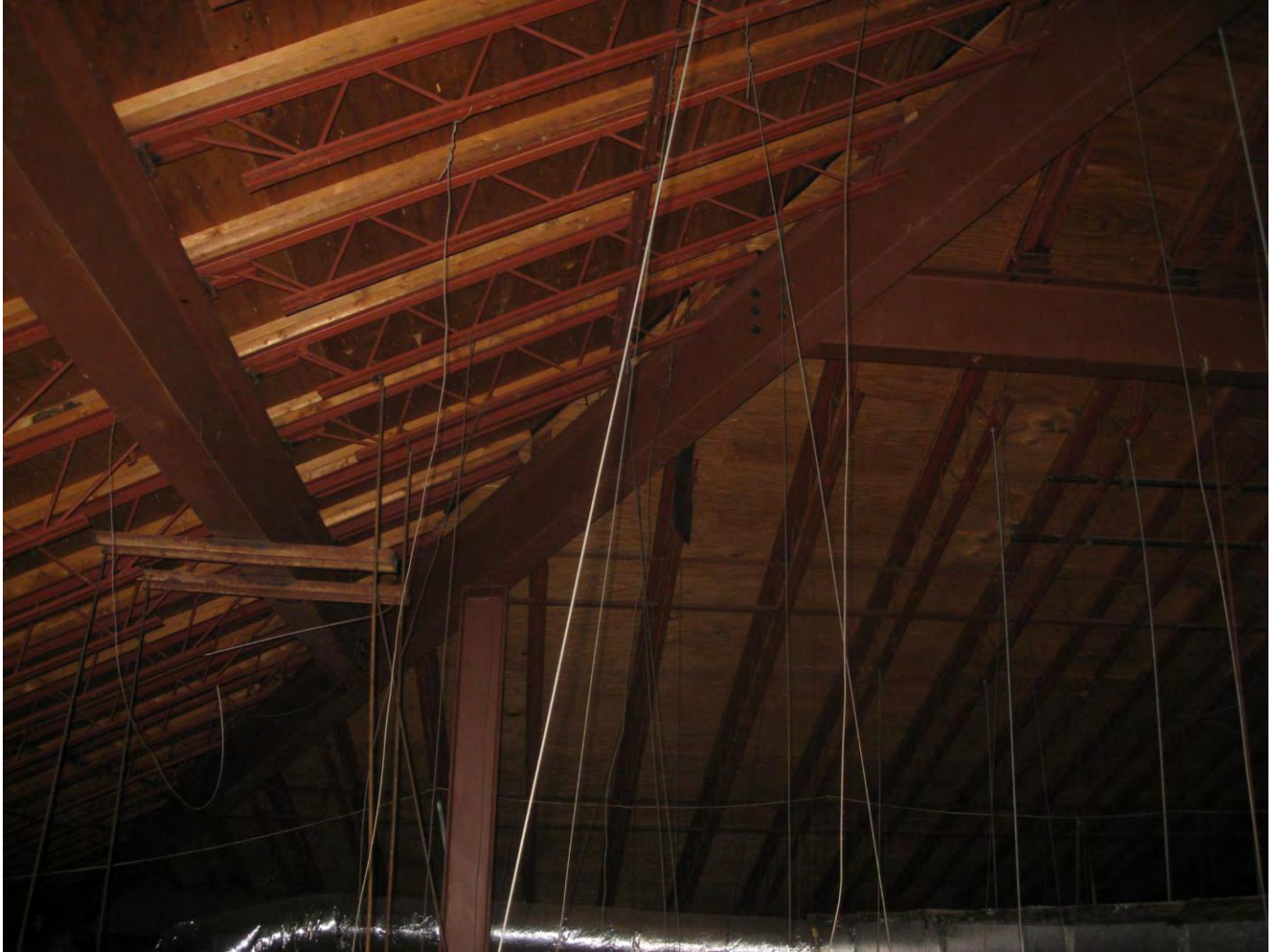
Picture 6: Portion of the steel column, beams and joists forming the hip roof structure.
