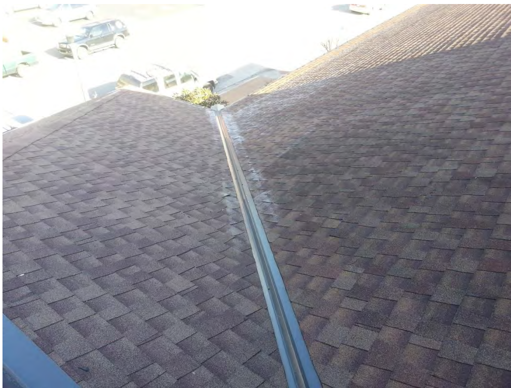
Valley metal pulling up from roof deck.
