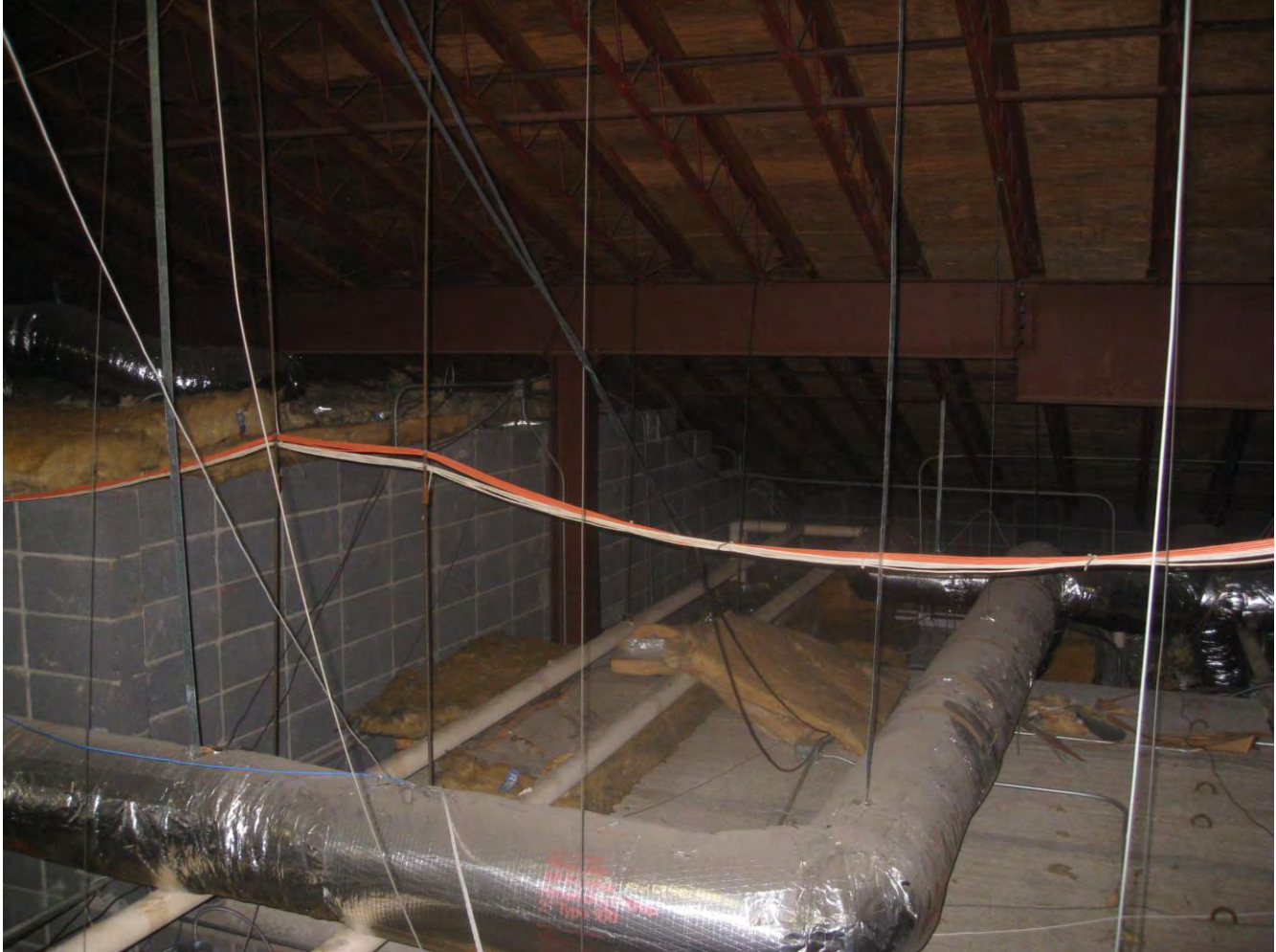
Picture 5: Steel joist and beam roof structure; no lateral support for the steel column or beam, and no concrete slab on deck for attic floor in this area.
