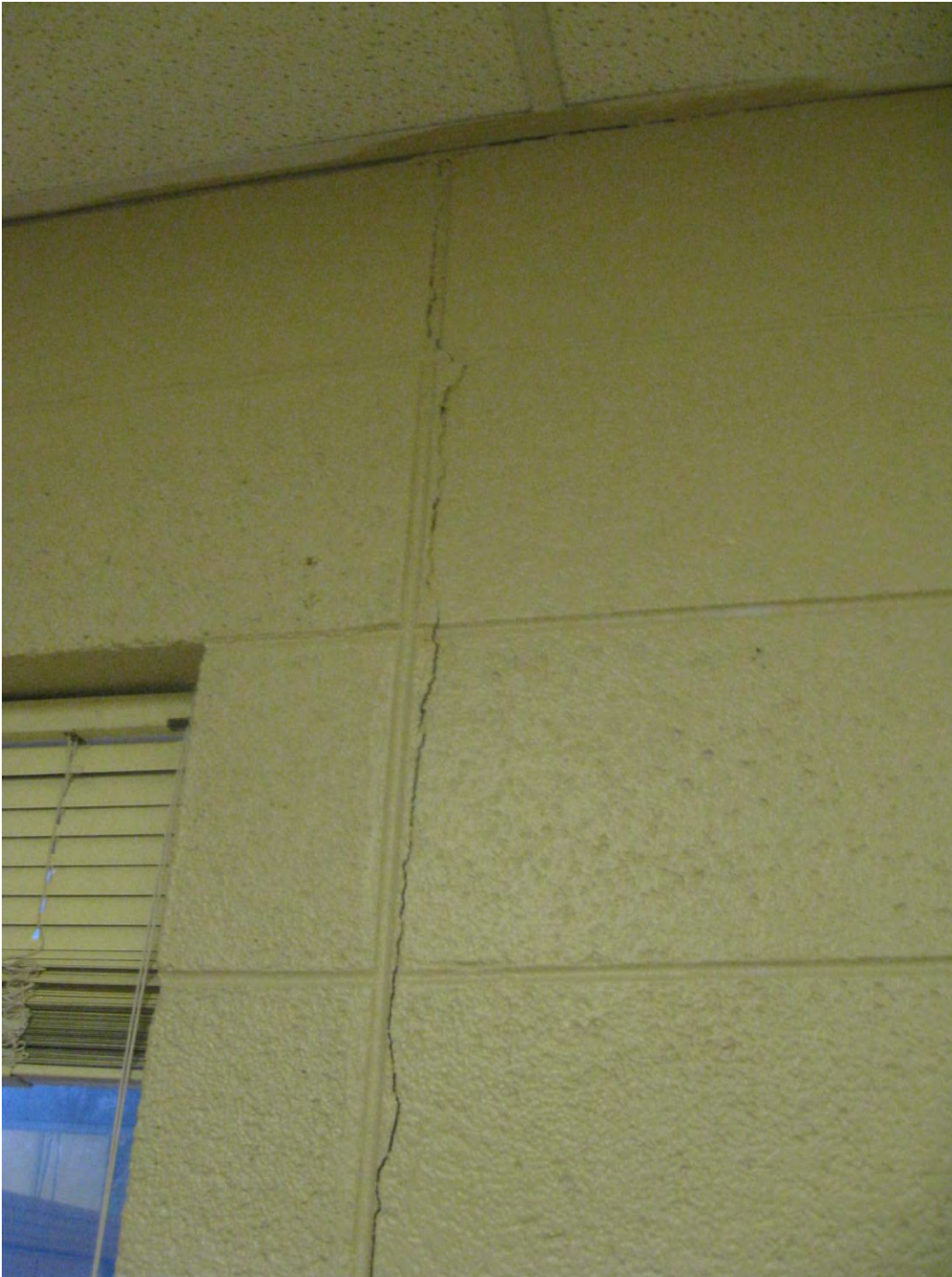
Picture 7: Vertical crack in an exterior masonry wall on the south side of the original building.
