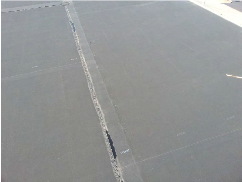
Seams beginning to curl and adhesive deteriorating.
