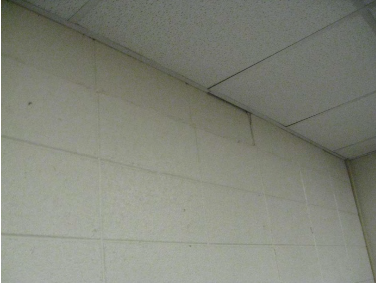
Picture 4: Displaced section of stack-bond masonry at top of exterior wall.
