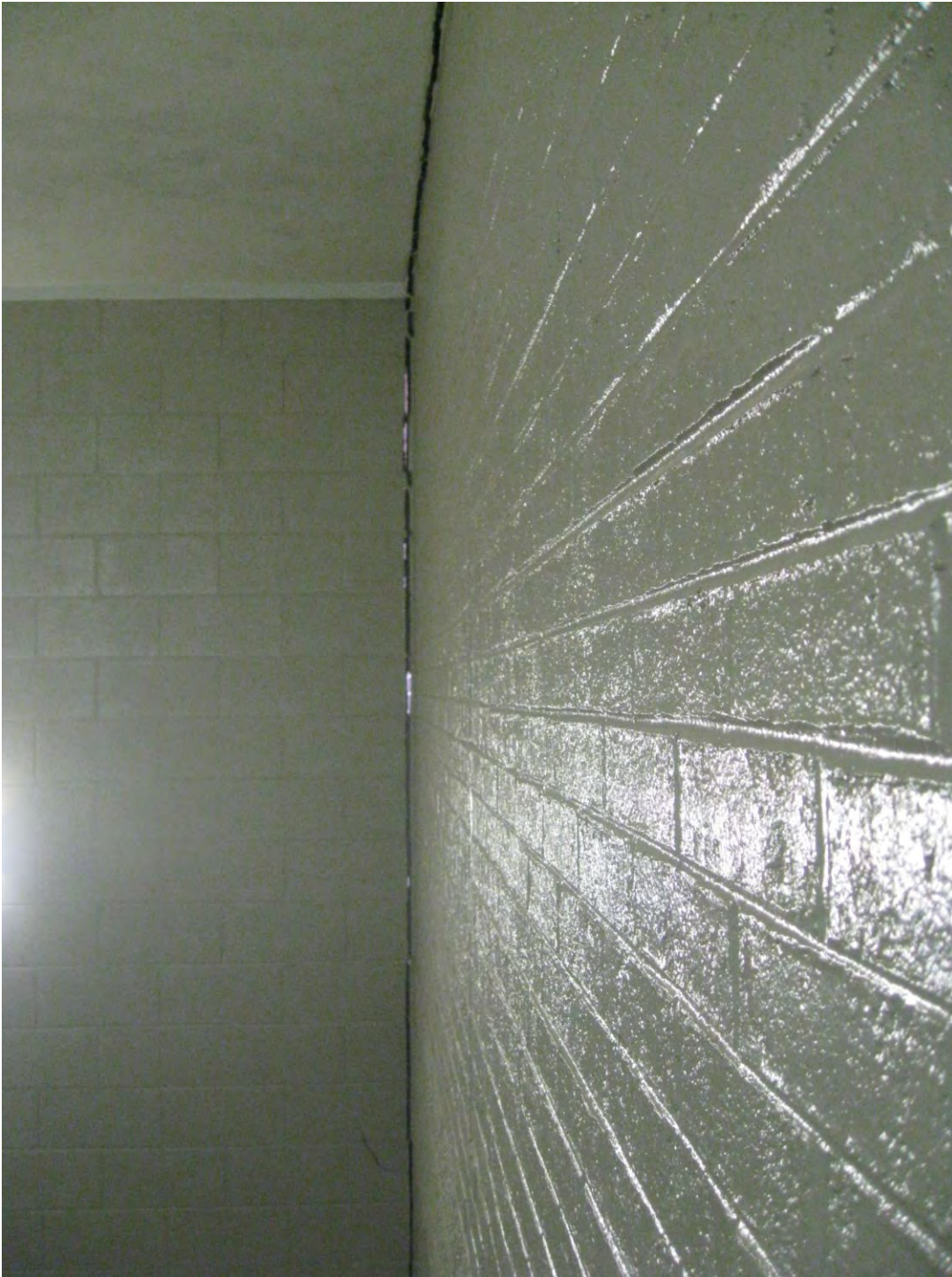
Picture 10: Separation of the newer stairwell wall from the Justice Center addition.
