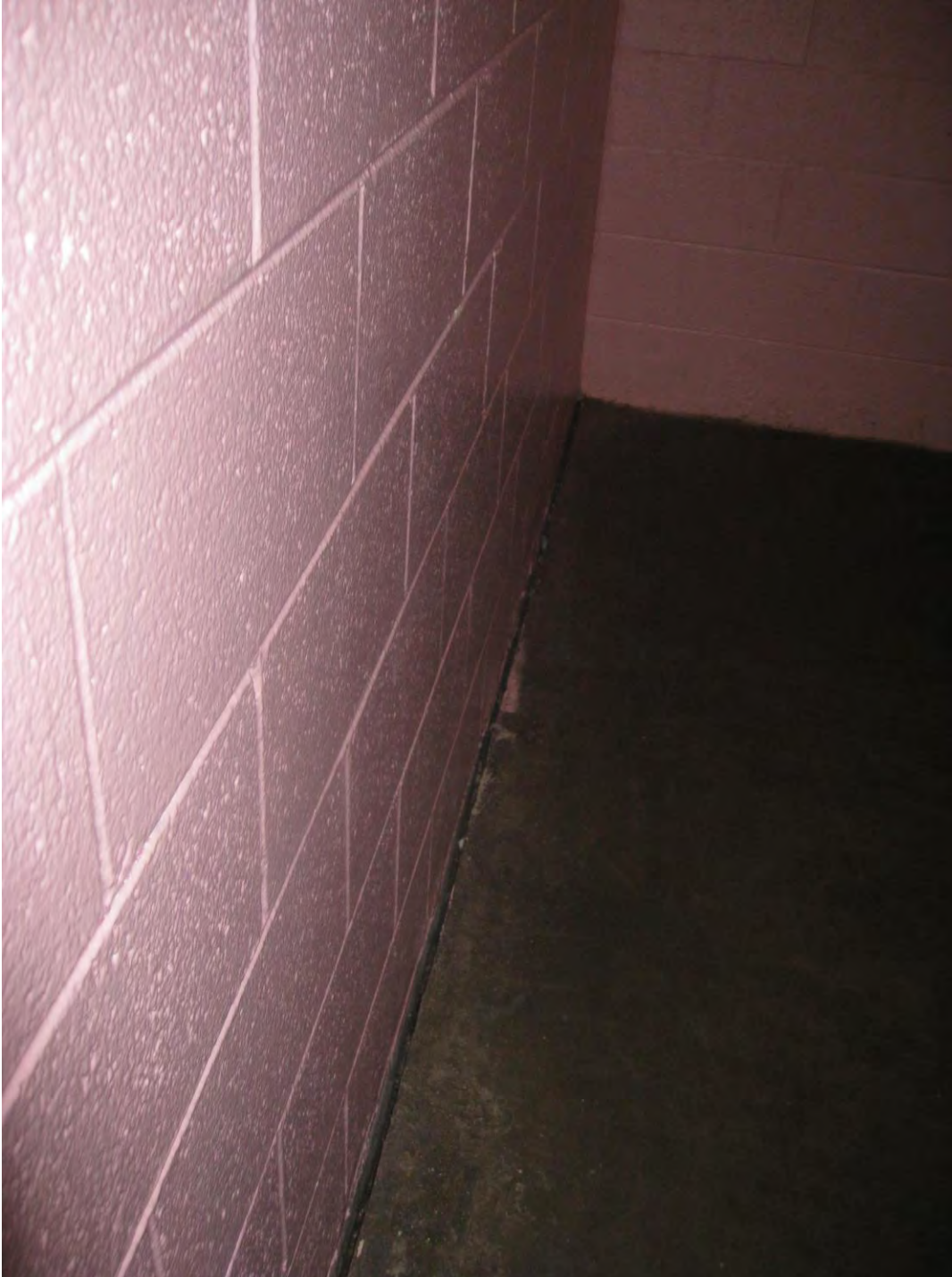
Picture 8: Separation of floor slab from exterior wall in the drunk tank.
