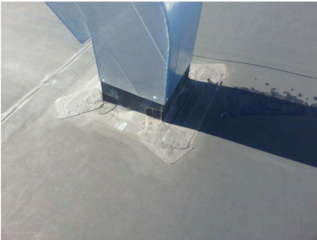
Flashing in good condition.
