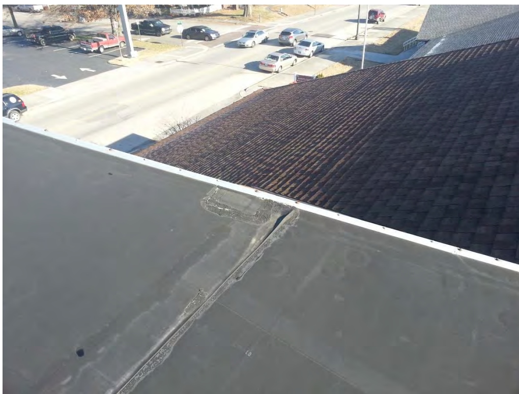
Seams beginning to curl and adhesive deteriorating.
